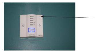
Immersion Heater, located above the sinks in the kitchen. This operates in the same way as the heater in the Main hall but will switch on the hot water immersion heater for the whole building (excluding the changing room showers).
